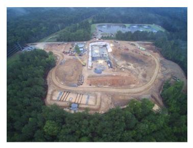
The above photograph gives an aerial view of the entire construction site, including the existing lagoon in the top right of the picture. The bottom left near the tree line shows a temporary water quality basin, which detains rain water runoff and prevents sediment from being dumped on to adjacent properties. Once construction is completed and the finished grades have been established, the site will be seeded to provide permanent stabilization to prevent erosion of the soil.
